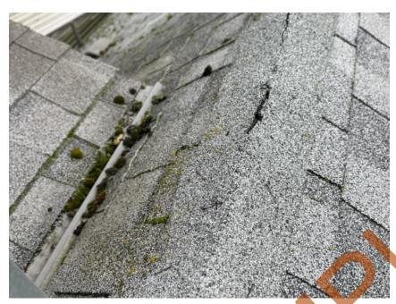
One cracked shingle observed at the ridge line near the roof peak. Likely due to age-related wear and prolonged UV exposure. While currently isolated, ridge shingles are critical for shedding water off the roof's highest point. Recommend replacing the damaged shingle to prevent potential moisture intrusion and further deterioration, especially given the roof's overall age.
