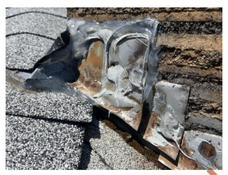
Chimney flashing is visibly deteriorated and improperly installed, with multiple cracks, corrosion, and excess sealant used as a temporary fix. These gaps create vulnerabilities where water can penetrate beneath the shingles and cause interior damage.
