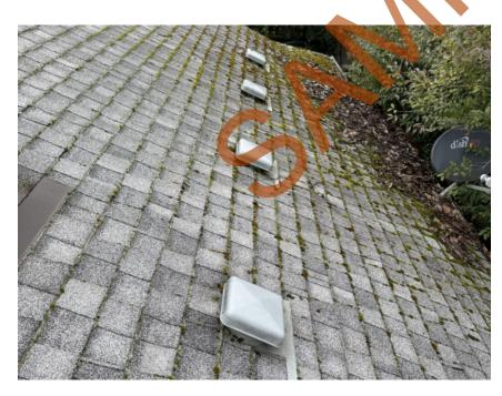
Significant moss growth and organic debris observed on the roof surface, particularly concentrated near the eaves and vents.
